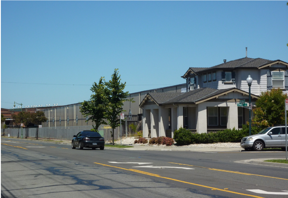
a) Oblique view of project site as viewed from Buena Vista Avenue at Ohlone Street.
