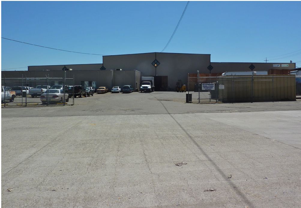
b) West end of project site as viewed from Entrance Road.
