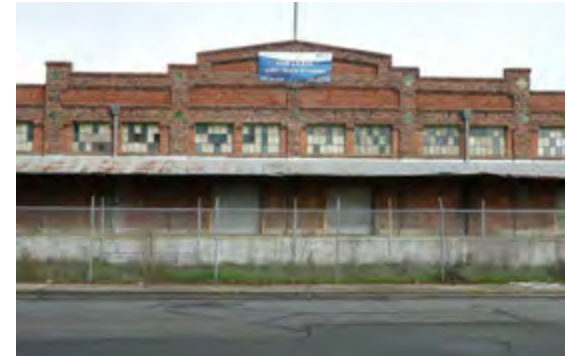
VIEW 4 - EXISTING CONDITION VIEW OF ENTRY ALONG BUENA VISTA AVE
