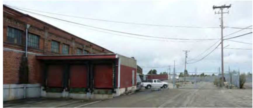
VIEW 2 - EXISTING CONDITION VIEW FROM ENTRANCE RD AND CLEMENT ALONG BUILDING FACADE
