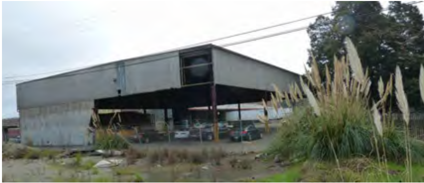
VIEW 1 - EXISTING CONDITION VIEW FROM SHERMAN ST AND EAGLE AVE
